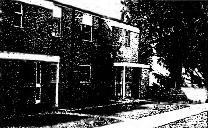
Kingston, Architect: Property Services Agencies, DOE.
